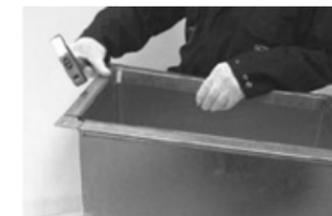
3. Fix completed SAF Flange frame at corner of duct section.
