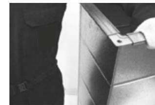
4. Corner of duct section must clear SAFID Corner Piece.
