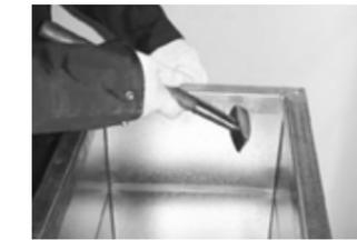
5. If duct section Corner is not clear tap the frame outwards to allow duct section to clear and slide past the SAFID Corner Piece.
