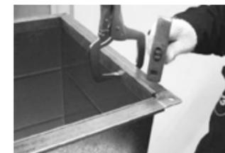
7. Establish metal to metal connection along the full length of the slide on flange.
