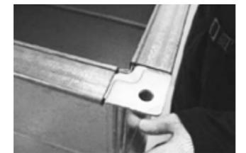
6. The duct section must be seated to the SAF - 35 so that leading edge of the duct section penetrates the mastic sealer. The corners of duct section should project above SAFID Corner Pieces.
