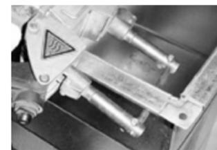
10. Fix and move in one direction around the duct flange. Do not attempt to fix flange at corners first, it could cause location problems.
