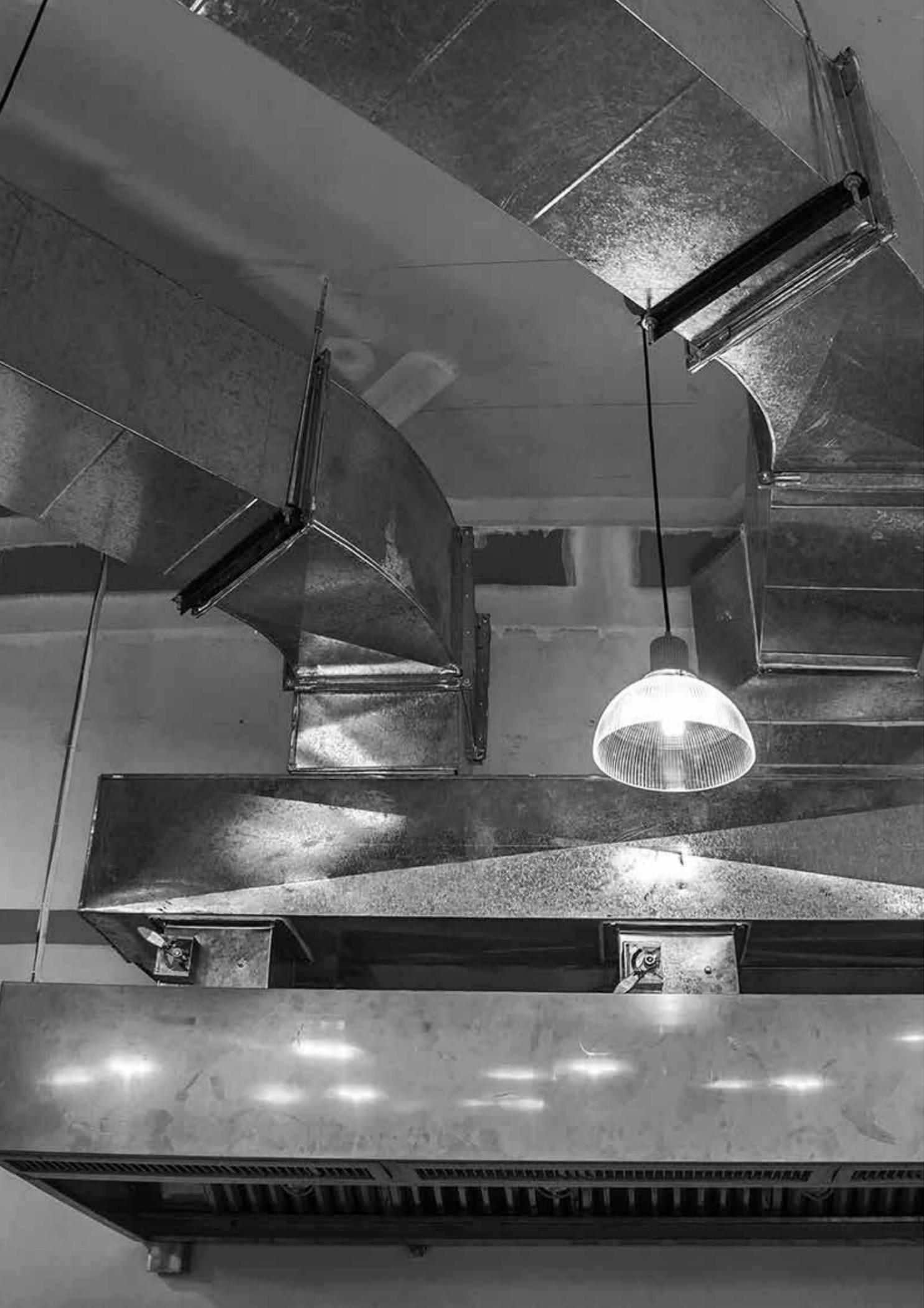
As the convection flow rises from the cooking equipment's surface, it expand in a certain degree angle. To be able to capture by the exhaust hood the expanding convection flow, the hood must be extended on all open sides beyond the cooking
